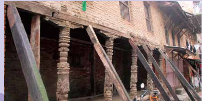
Beams support houses that wait to be reconstructed in Kathmandu.
